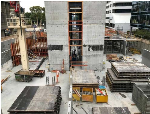
Fig. 2: Formworks to Level 1
