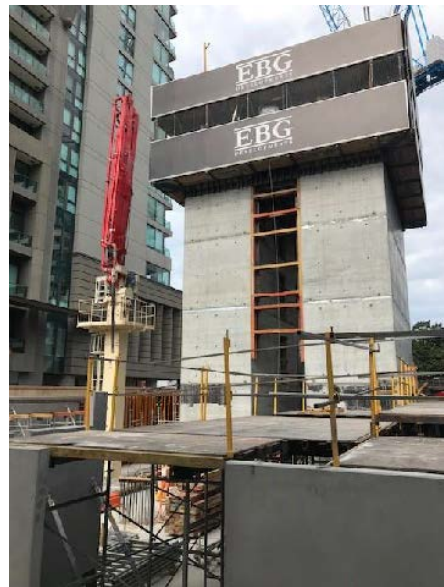
Fig. 3: Lift core Structure
