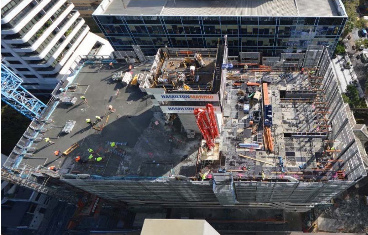
Fig. 1: View from Top – Constructing Lift Core & Slab
