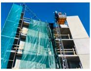
The crane is scheduled to be removed from the site in the upcoming weeks and the mobile hoist has been mounted to the front of the building to deliver the materials to each floor. The BlueScope steel frames have been sitting on the top floor ready to be assembled finalizing the 4th floor structure.
