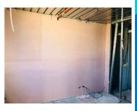
Metal and timber framing inside the apartments is in the process of being completed. The pink fire rated shaft liners have been installed as partiwalls between apartments along with earth wool insulation. The silvery insulation boards have been attached to the concrete walls, framed, cabled and plumbed for fit off once the joinery arrives.
