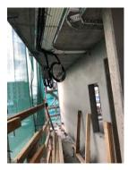
The dark red metal plumbing of the fire sprinklers indeed makes a statement and provide a contrast to the yellow gas pipe lines sitting in unison in a cable tray. These trays make way to the north face of the building in the service cupboards neatly tucked behind the façade along with other infrastructure equipment i.e. gas meters, water check meters, NBN cabling etc.
